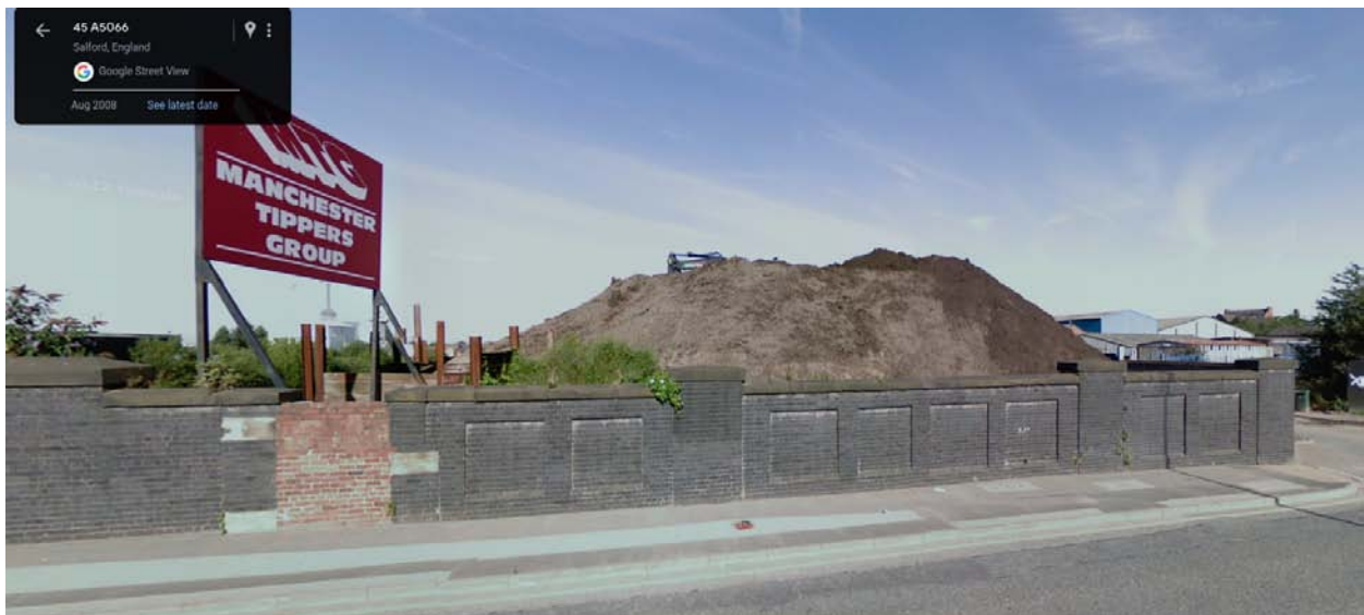
View taken in 2008 of the heritage canal bridge parapet showing the bricked up access to the original towpath (source: Google Street View).
