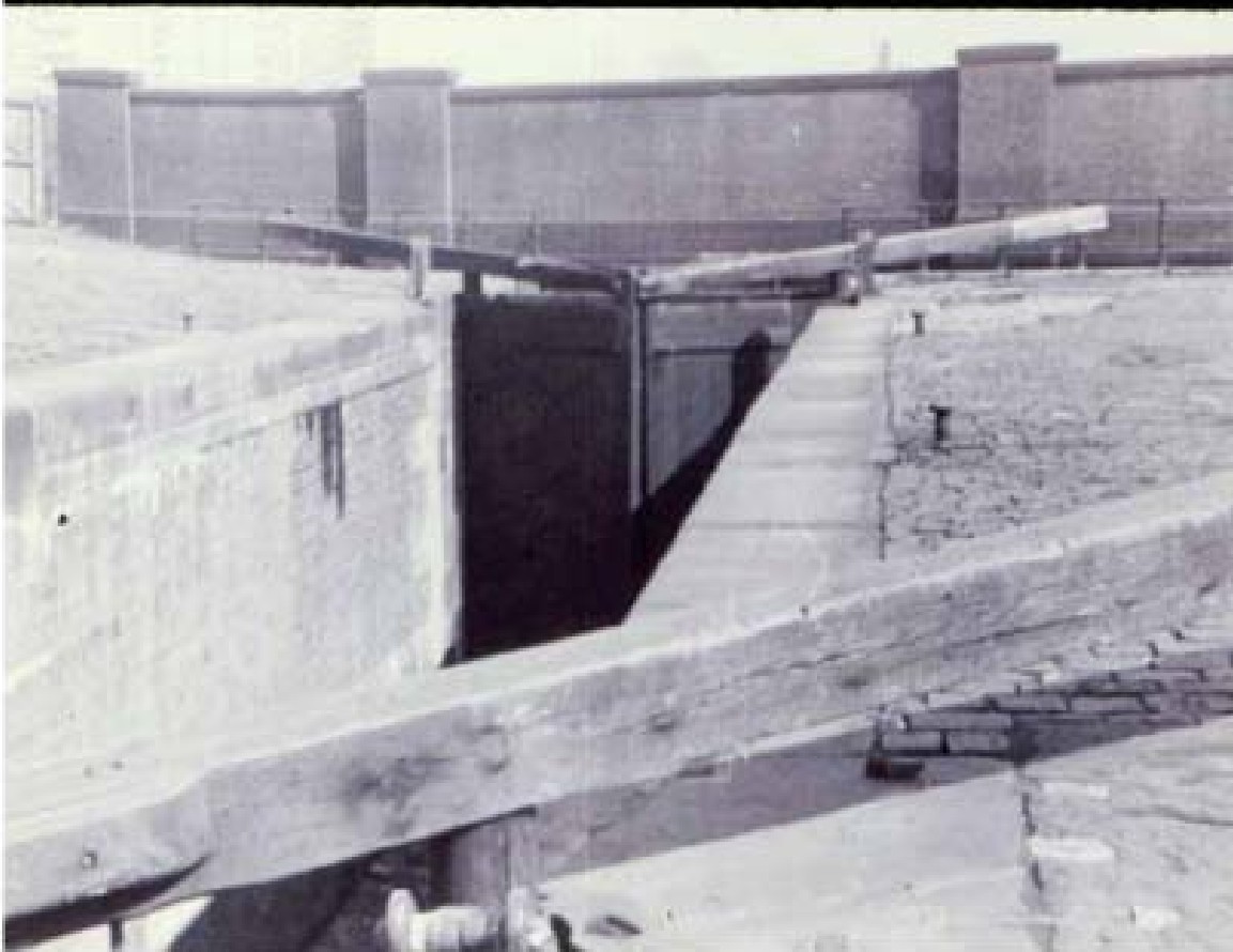
Lock 5 Head Gates - view towards Oldfield Road
